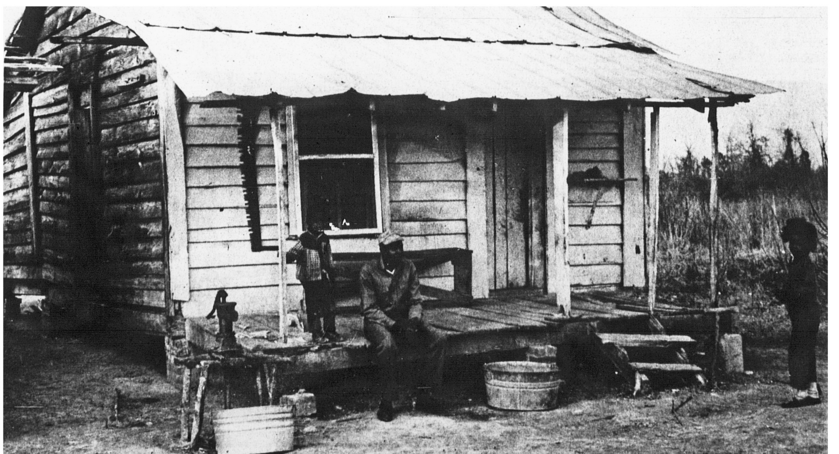
CHARLES WASHINGTON'S CABIN HAS WHITEWASH BUT NO HEAT, LIGHTS, OR WATER
