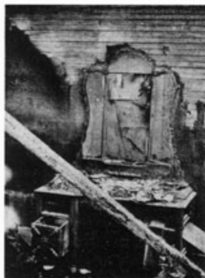
AFTER THE FIRE
