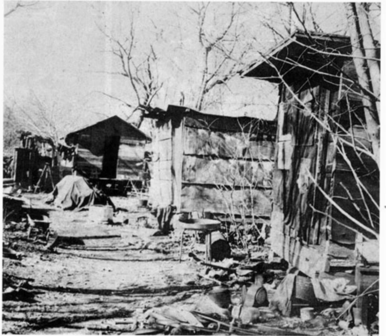
"THE DITCH" IN NORTH MOBILE
