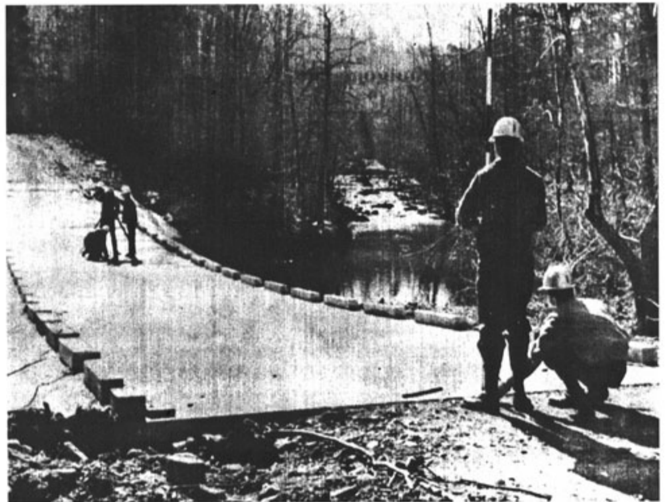
JOB CORPSMEN SURVEY ROAD IN ARKANSAS
